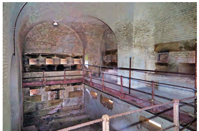
Caponier interior, original slanted musket embrasures above, WWII era firing slots below right, the carronade embrasures bricked up. Photo Clive Penfold
